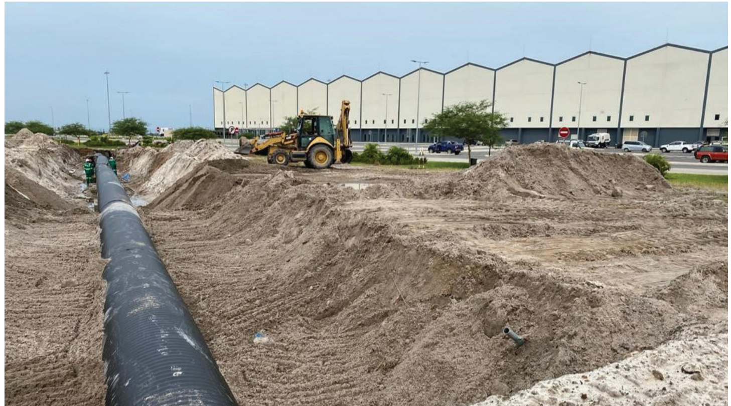
Stormwater Drainage (Stormwater drainage line for Julius Nyerere International Airport, Terminal 3).
