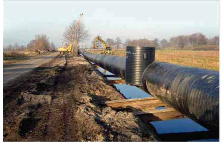
Discharge pipes for waste water treatment plant
