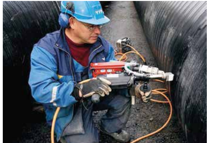
Hand-held extrusion machine. Hand extrusion is especially suited for waterproofing thread joints
